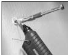
Losse deuvels vastzetten.
