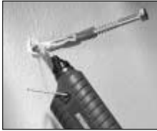
Securing loose wall plugs.
