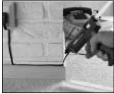
Laying telephone cable.
